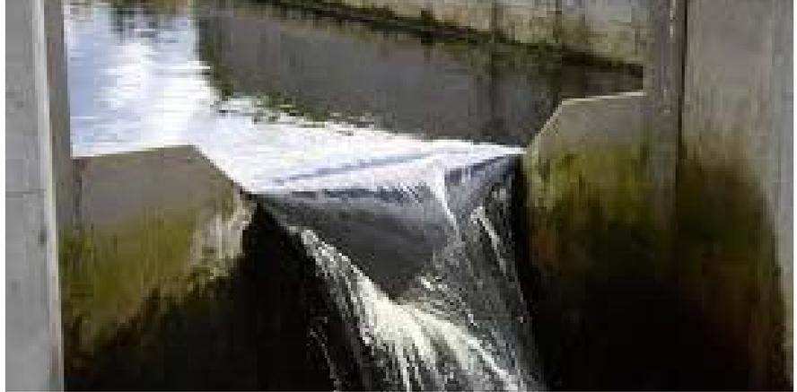
Typically installed in open channels, the function of a V-notch weir is to determine discharge (flow rate) from a body of water, such as a dam or stream.
